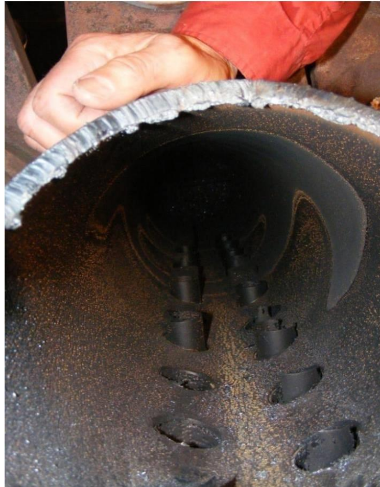
2011 view of FAC damage before header replacement
