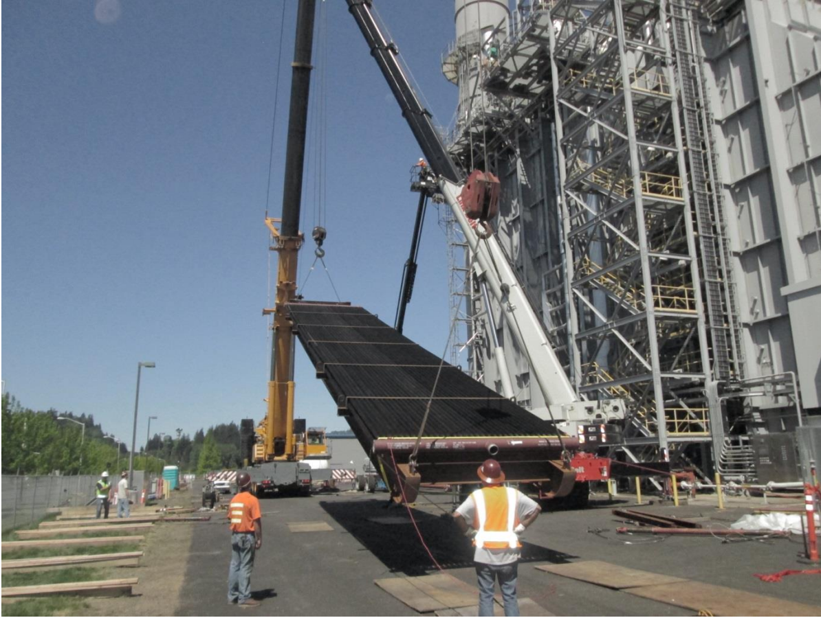
Replacement HRST Shockmaster® economizer bundle
