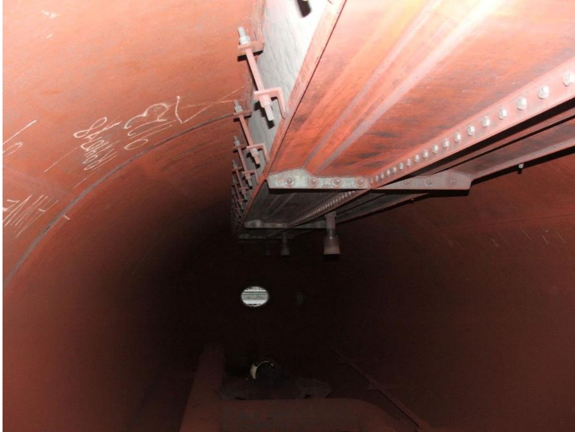
Drain Traps in place
