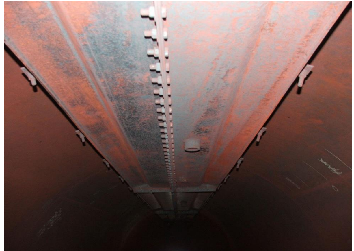
Drain Traps missing
