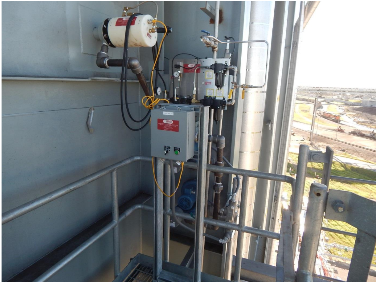
Duct Burner Camera for Control Room Viewing
